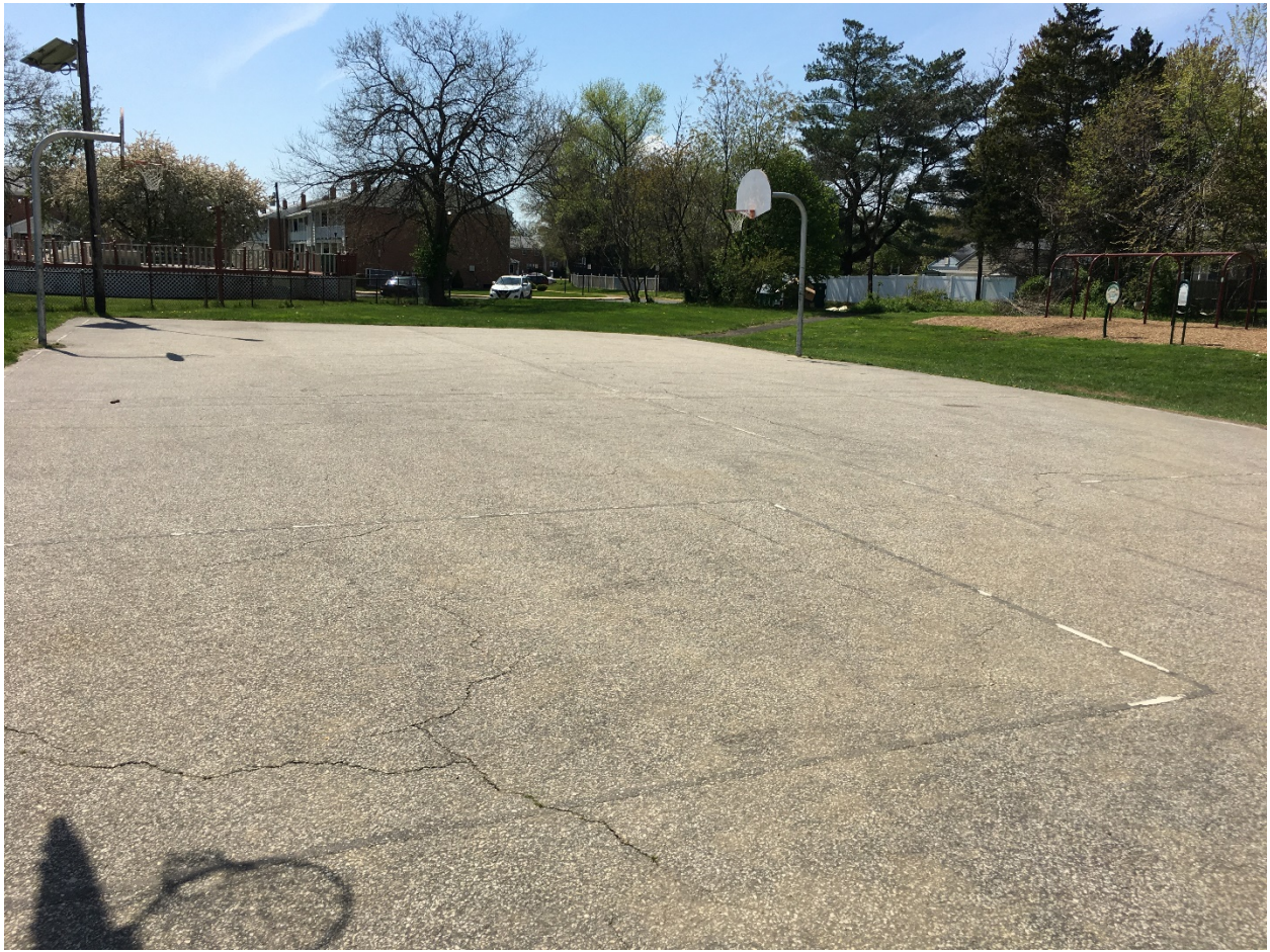
London Square Park – Basketball court with evidence of cracking
