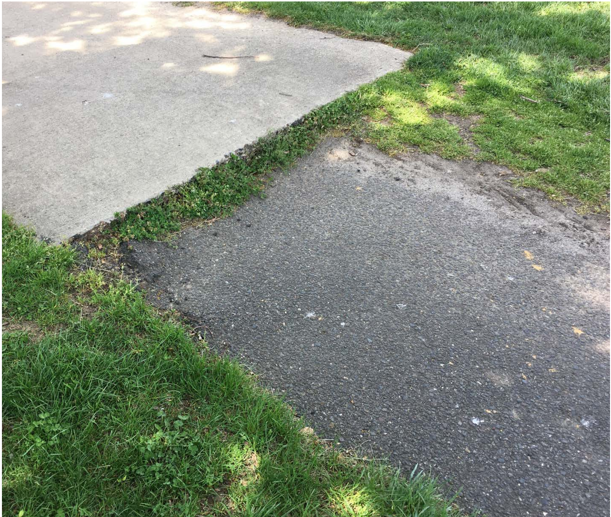
Green Lane – Walking path, note variety of surfaces and levels, trip hazards and lack of ADA access
