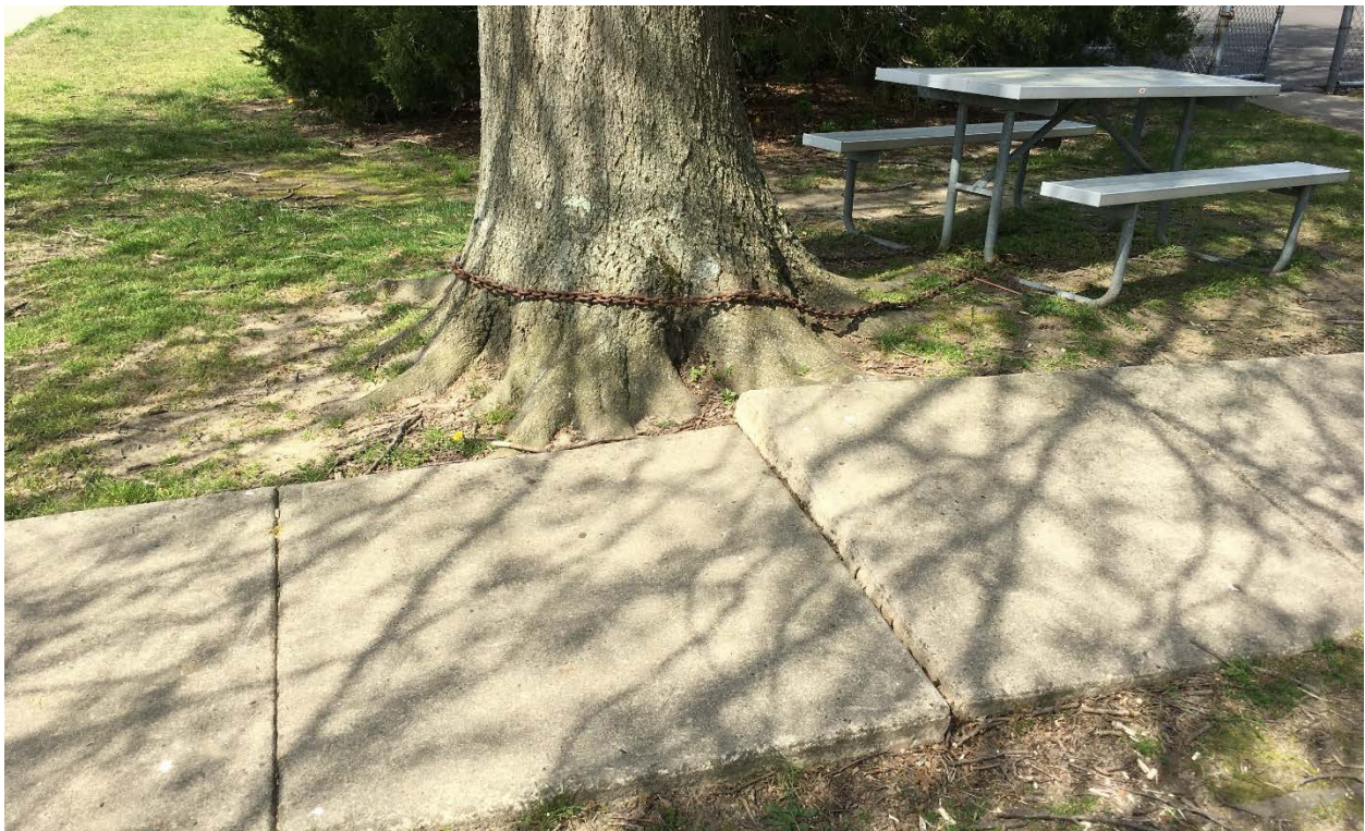
Glen Eayre – Note sidewalk heaving from tree roots
